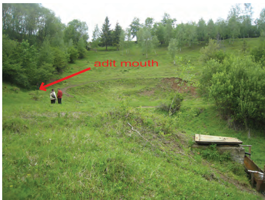
Fig. 6.10 Situation of caved-in adit collar of Všechnsvätých Gallery in Rudňany prior to its opening and reconstruction.
