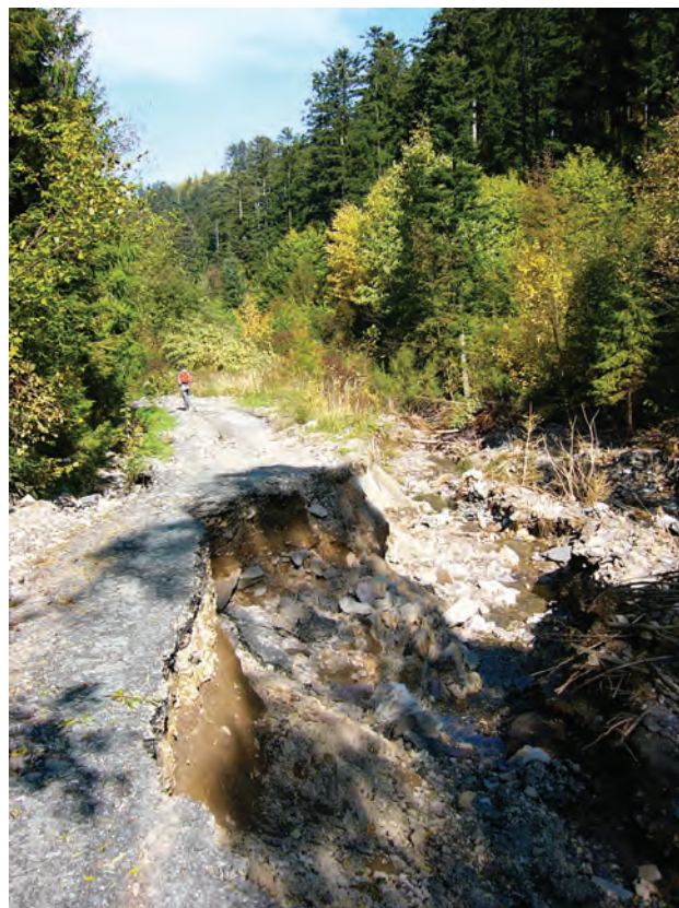
Fig. 6.7 Local road eroded by flood wave of mine water inrush from Nová Gallery (photo Baláž)
