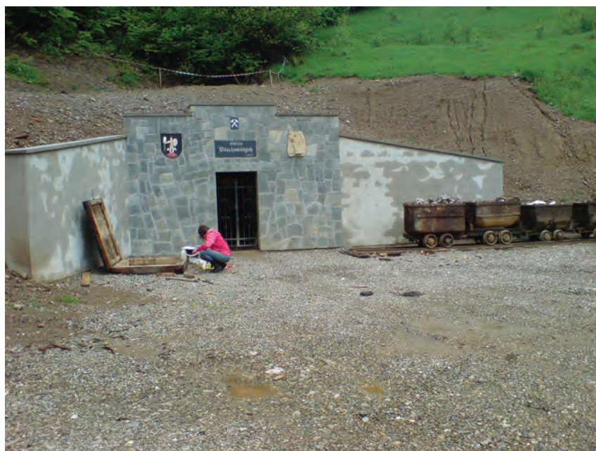
Fig. 6.11 Portal built in 2013 at former caved-in adit collar of Všechnsvätých Gallery in Rudňany
