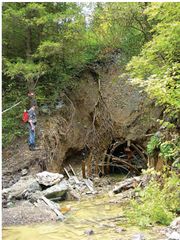
Fig. 6.6 Mouth of Nová Gallery destroyed by mine water inrush from abandoned mine (photo Baláž).
