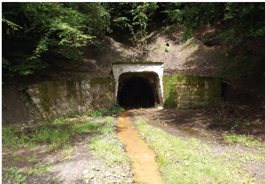
Fig. 6.8 Mouth of Budúcnosť Gallery near Pezinok with mine water discharge with precipitating Fe-ochre (photo Baláž).
